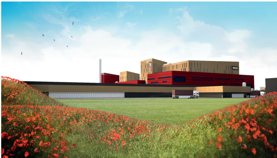
NW Corner Site Boundry
